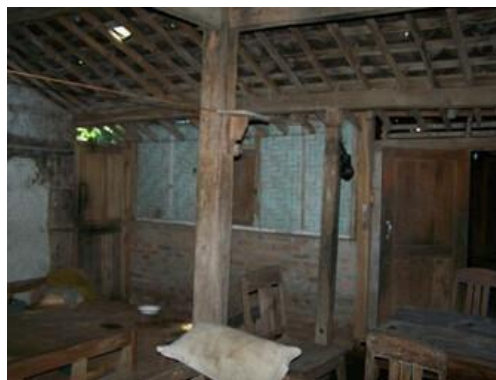
Figure 2. Interior structural elements of Rumah Sandi Dukuh, showing timber columns and roof framing Photograph by the author, Dusun Dukuh, Samigaluh, Kulon Progo, 24 September 2024. Reproduced by permission of Museum Sandi.
